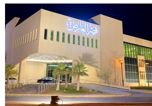
RRC Qasr Alaaredh Company Project Building
