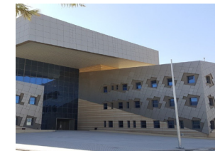
جامعة المعرفة ALMAAREFA UNIVERSITY Almaarefa University Project Building project
